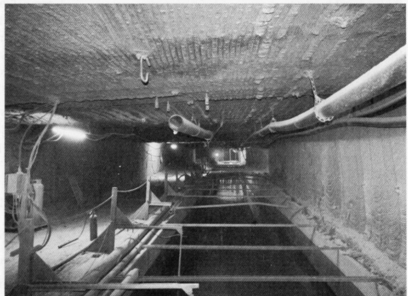
Saturated brine pumped from within the mine – Photo by Nick Catford
